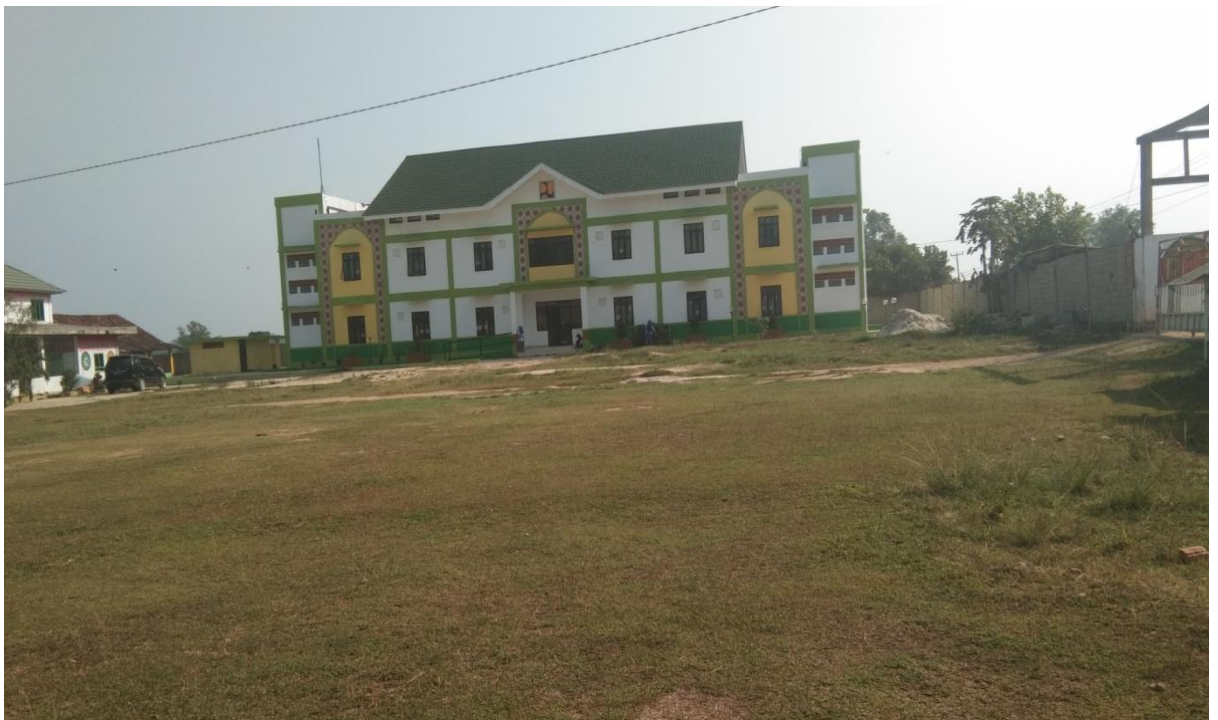
The condition of the Student's Dormitory
