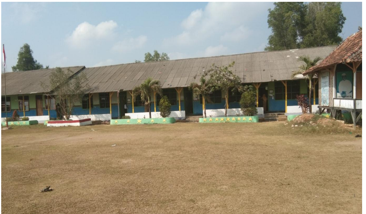
The condition of the Classroom
