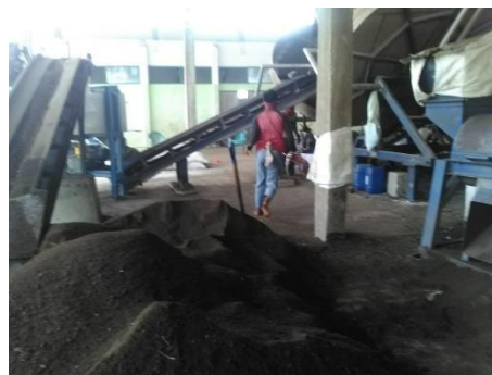
Gambar 4.1 Proses Penghalusan (Crushing)
