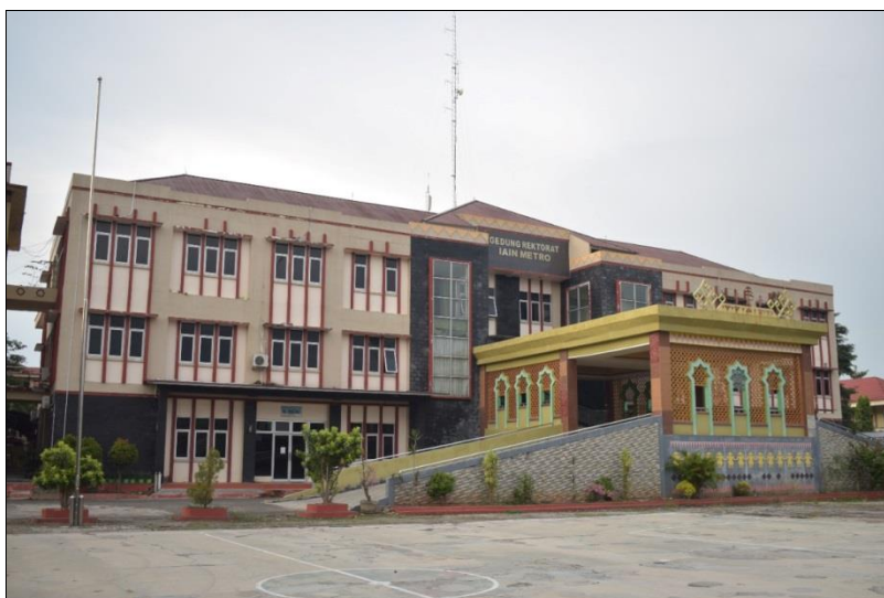
Picture 4.1 Building of IAIN Campus 1
