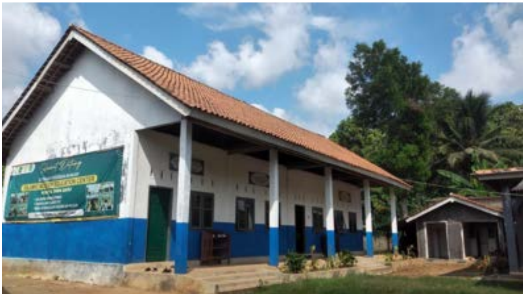
Building Condition of SD Islam Modern An-Najah Sambikarto
