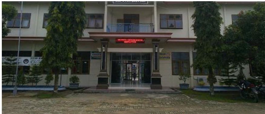
Picture 4.1 SMK Insan Cendikia Building
