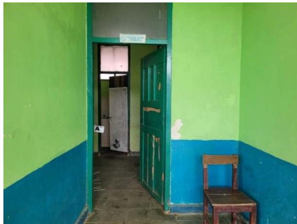
Toilet wanita SMAN 1 Purbolingo
